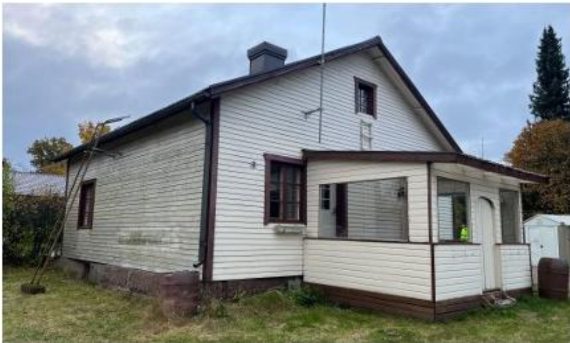
Figure 14. The demolition site is a 1900s log-frame detached house. (Puutuoteteollisuus ry, Double Round Oy, 2025)
