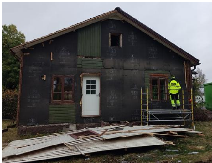
Figure 16. The outer exterior cladding (white) has been removed using excavator and laid on the ground (Puutuoteteollisuus ry, Double Round Oy, 2025)
