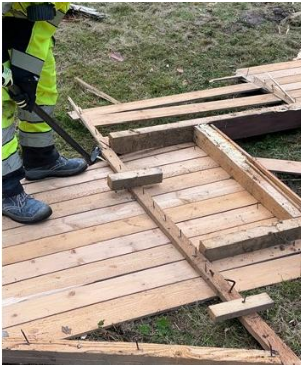
Figure 17. The dismantling was done by hand on the ground. (Puutuoteteollisuus ry, Double Round Oy, 2025)
